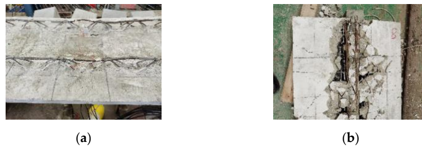
Figure 7. Specimen failure diagram: (a) Upper chord rebar crimping; (b) Concrete crushing.
