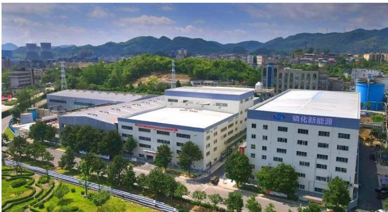
Figure 4. The new energy plant of the Guizhou Phosphate Chemical Group.
