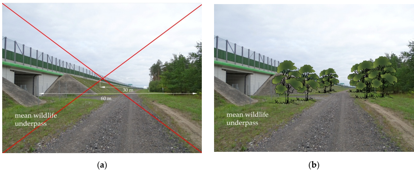
Figure A10. Landscape and land development features in the surroundings of a medium underpass: (a) Poor land development around a stream, one-year-old tree seedlings planted after the road was open for traffic, inadequate for the altitude of bat flight and the inside clearance distances of the underpass, absence of a screen raising the height of bat flight; (b) Proposed installation of a mesh screen and planting of mature trees adequate for the height of bat flight and the inside clearance distances of the wildlife underpass, directed straight at the wing walls of the underpass.
