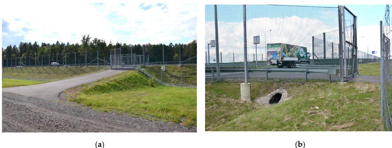
Figure 10. Exit gate on the expressway section with mesh screens: (a) Ramp off to the service road; (b) Safety mesh netting on the exit gate.
