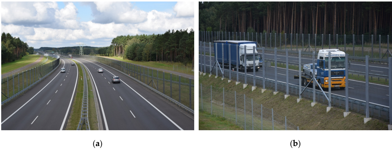
Figure 8. Structural details of mesh screens: (a) View of the S3 expressway with mesh screens on both sides; (b) Steel posts with braces.
