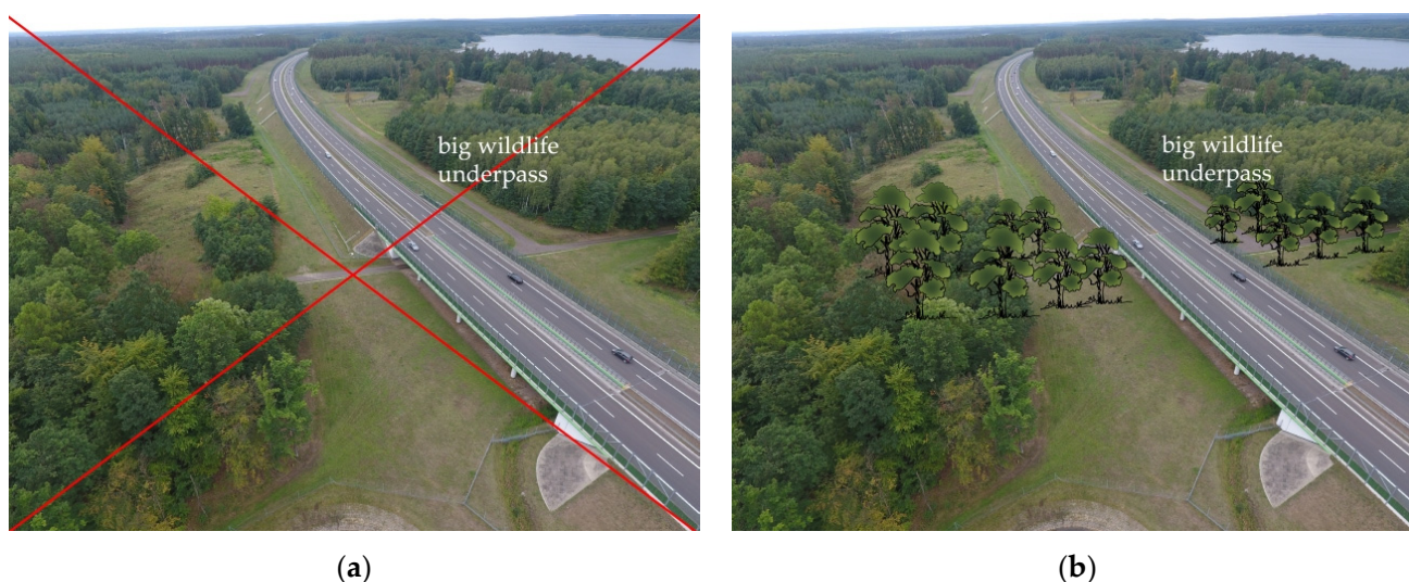
Figure A11. Landscape and land development features in the surroundings of a large underpass: (a) Poor land development around a stream, one-year-old tree seedlings planted after the road was open for traffic, inadequate for the altitude of bat flight and the inside clearance distances of the underpass, absence of a screen raising the height of bat flight; (b) Proposed installation of a mesh screen and planting of mature trees adequate for the height of bat flight and the inside clearance distances of the wildlife underpass.
