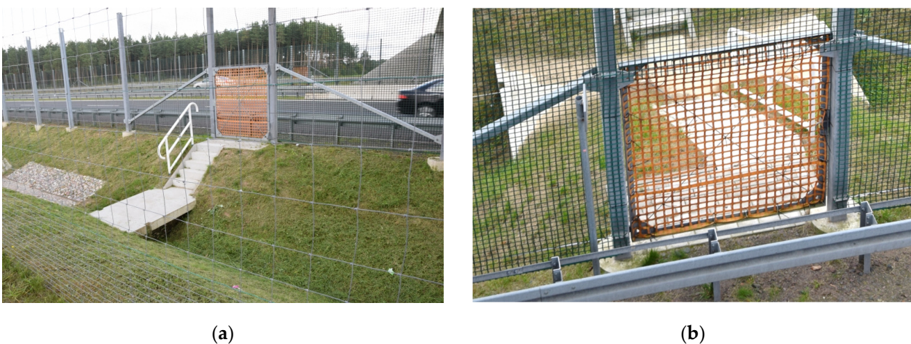
Figure 9. Emergency exit: (a) Stairs and landing to allow evacuation of the road users in case of emergency; (b) Easily removable safety mesh netting at an emergency exit point.
