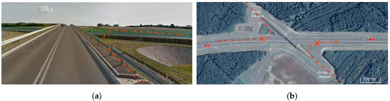
Figure 6. A hypothetical visualisation of a bat flight trajectory along the old route of a local road newly constructed on an overpass bridge over a newly completed dual carriageway: (a) View of a hypothetical bat flight route from the local road on the overpass bridge with no additional guiding elements; (b) Aerial view of a bat flight route along the overpass and further along the S3 expressway with mesh screens installed on both sides. (Visualization by the authors based on the description of the research and conclusions given in [76]).
