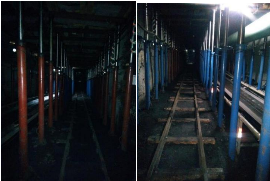
Figure 15. Support effect of the roadway.
