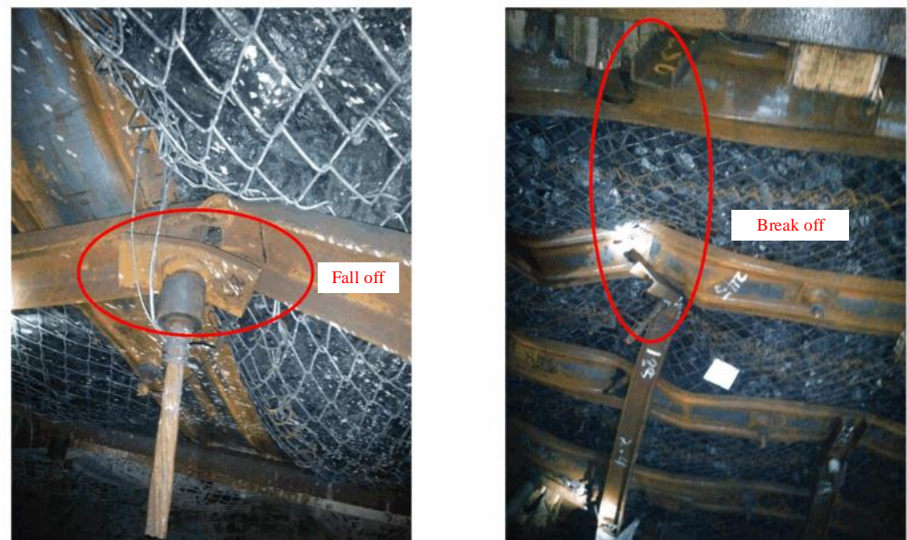
Figure 4. Diagram of field support failure.
