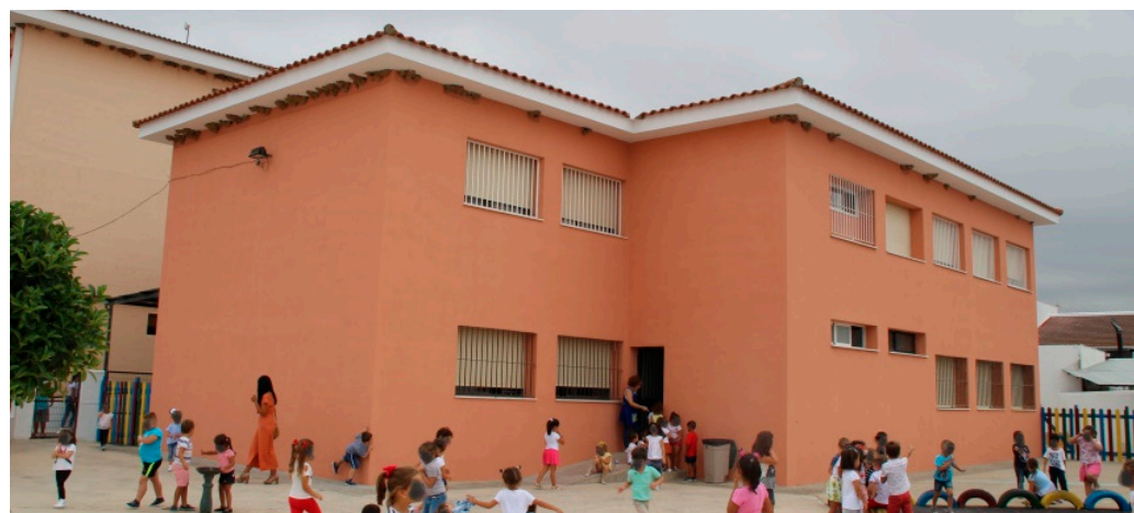
Figure 7. Long façade after retrofitting.
