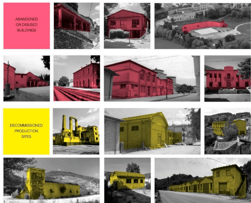
Figure 14. The spaces of possibilities, abandoned industrial sites, and productive heritage detected through a pattern analysis in the whole inner area. Credits: M.G. Di Baldassarre, 2022, ©Branding4Resilience—UNIVPM, 2020–2023.
