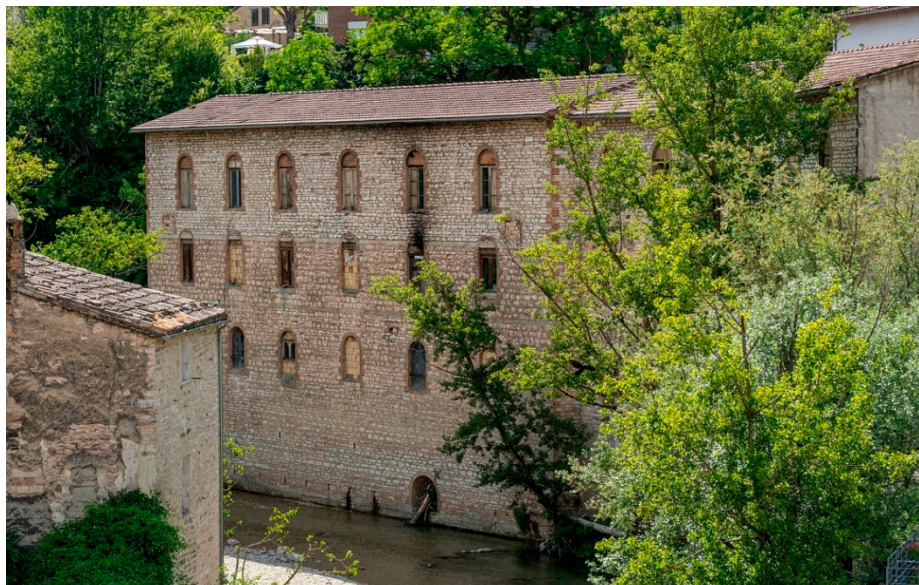
Figure 13. Former pasta factory Giacani next to the historical center of Sassoferrato (AN). Photo by A. Tessadori, 2021. ©Branding4Resilience—UNIVPM, 2020–2023.
