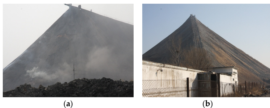
Figure 1. Photos of gangue piles in use in a coal mine area in Liaoning Province. (a) Gangue pile in spontaneous combustion; (b) gangue pile without spontaneous combustion.
