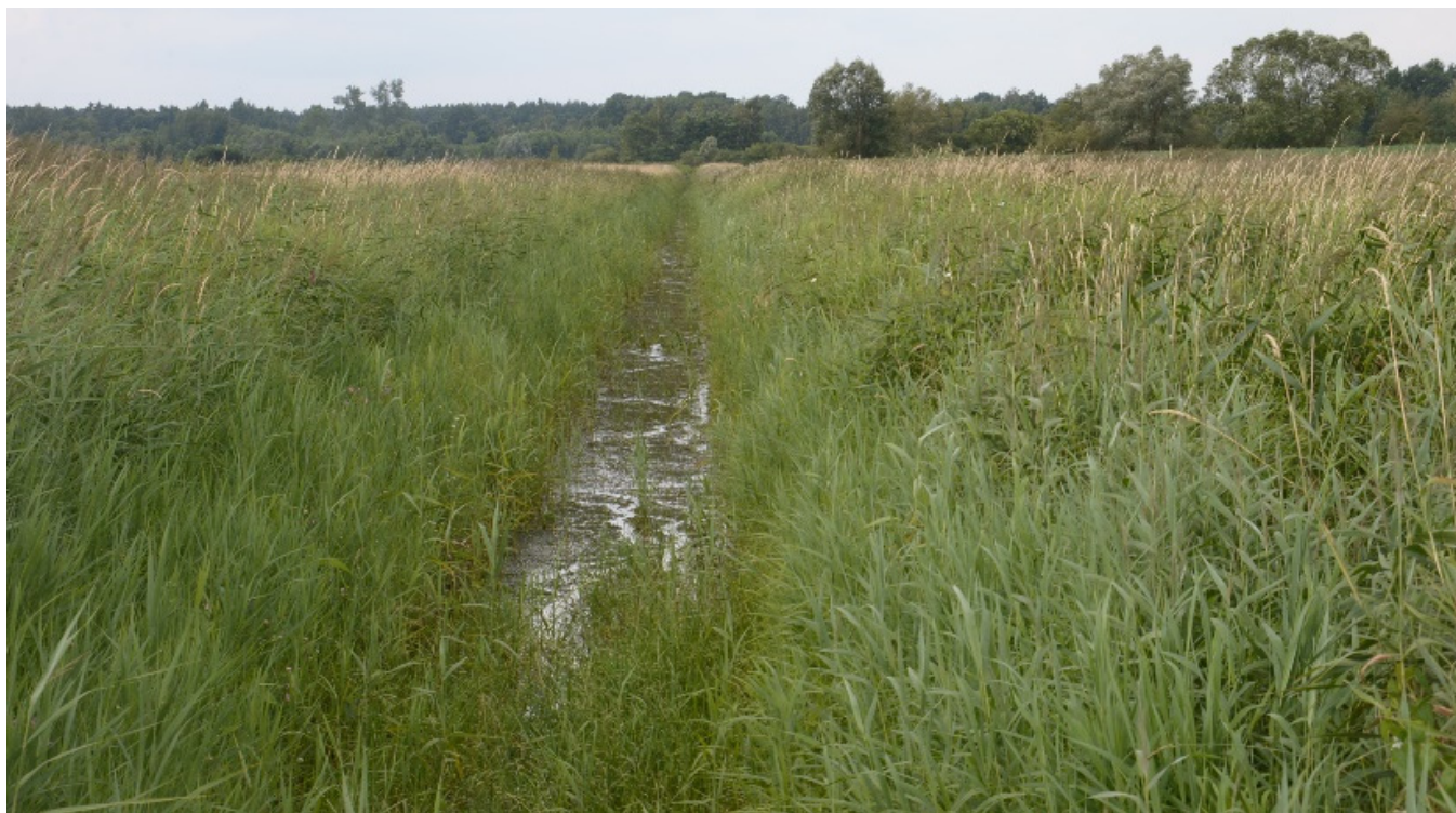
Figure 8. An example of poor maintenance of a drainage ditch in Strzelce Wielkie (photo: T. Wirth).
