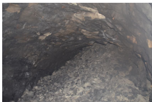
Figure 1. A photo showing the roof collapse of a mining tunnel in the fault fracture zone.
