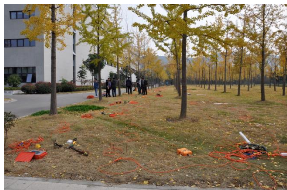
Figure 3. ERT instrument installation and electrode array installation.
