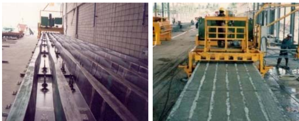
Figure 5. Long-line system method concrete placing.
