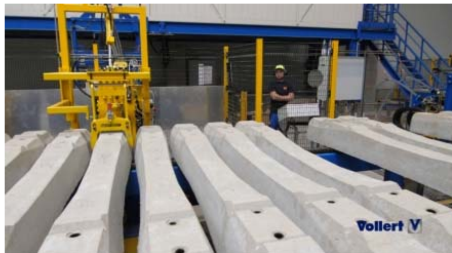
Figure 17. Post-tensioned short-mould flow method tensioning process.
