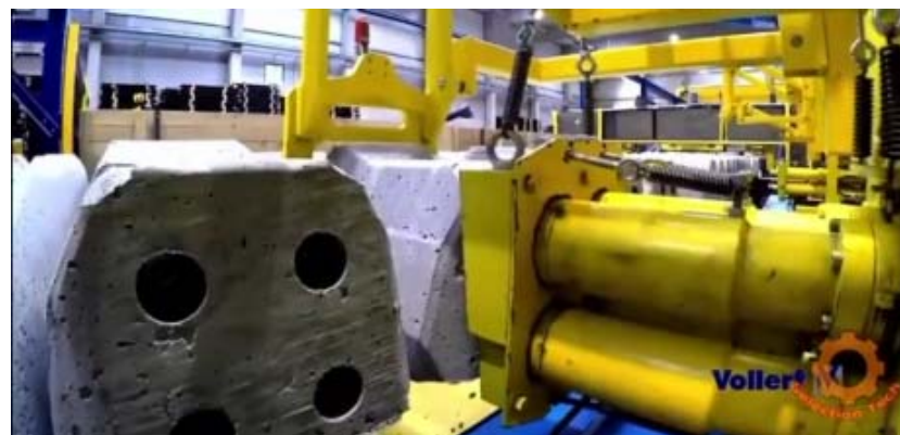
Figure 22. Tensioning and anchoring process of the instant-demoulded short-mould flow method.
