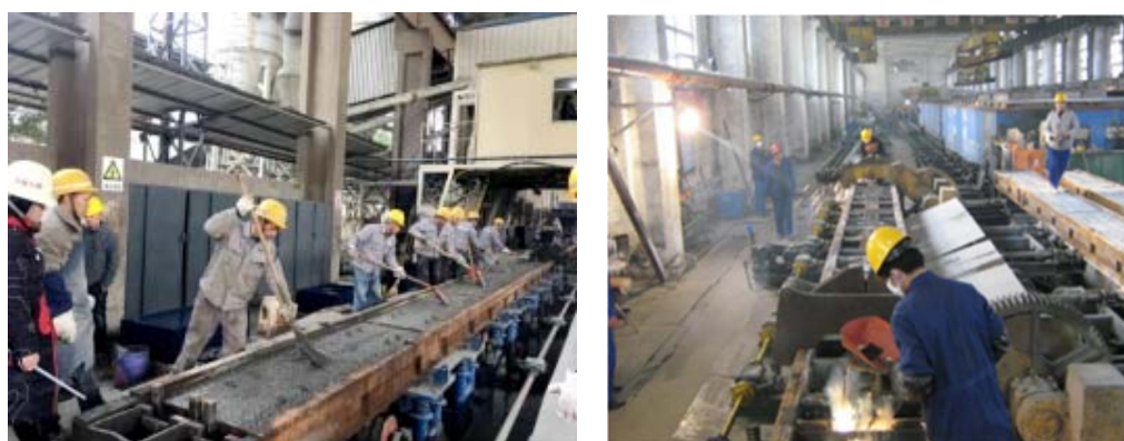
Figure 10. Concrete vibration and prestressed force transmitting of long-mould flow method.
