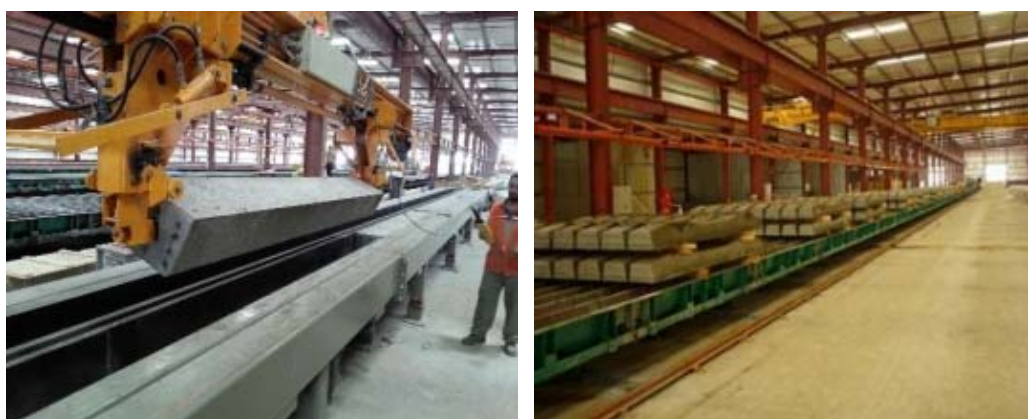
Figure 6. Long-line system method sleeper demoulding.
