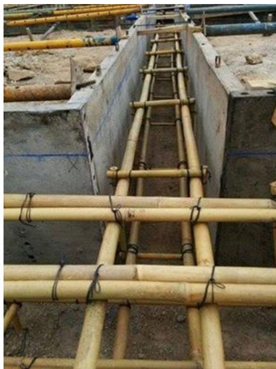
Figure 4. Bamboo in replacement for steel reinforcement.
