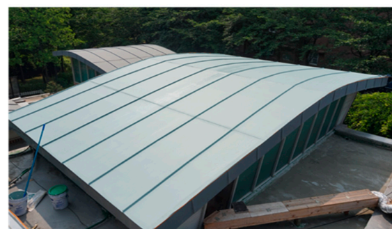
Application of cool roof coating
