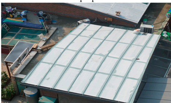
Reinforcement of vulnerable areas
