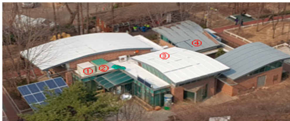
Figure 2. Bird's-eye view of the case study site (image source: authors). ① Experimental model (cool roof) ② Experimental model (Conv. Roof) ③ Actual Roof (Cool Roof) ④ Actual Roof (Conv. Roof).
