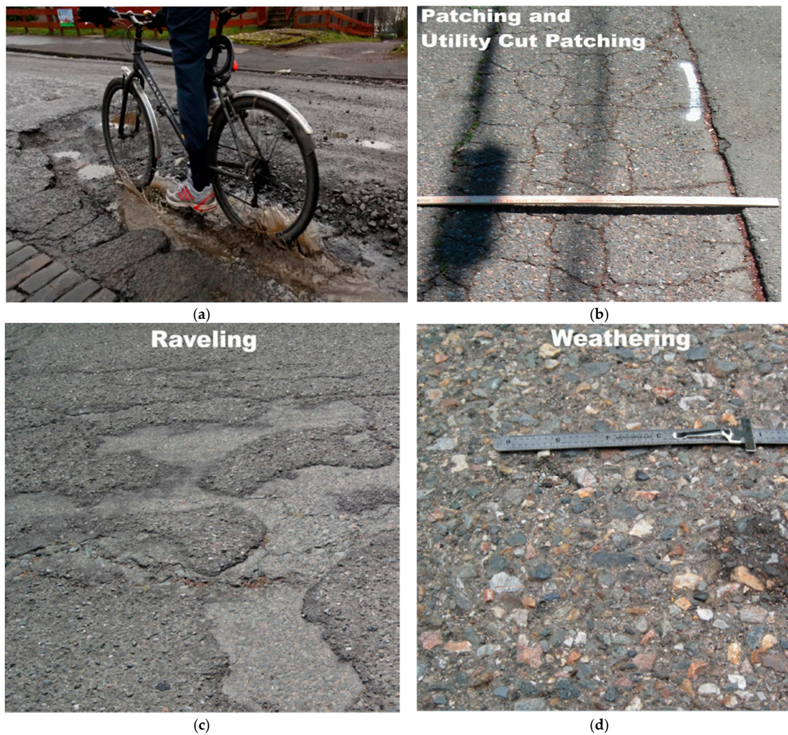
Figure 1. Examples of flexible pavement distresses affecting bicyclists: (a) Potholes [2]; (b) Cracking and Rough cut Utility Patching [3]; (c) Raveling [3]; and (d) Weathering [3].
