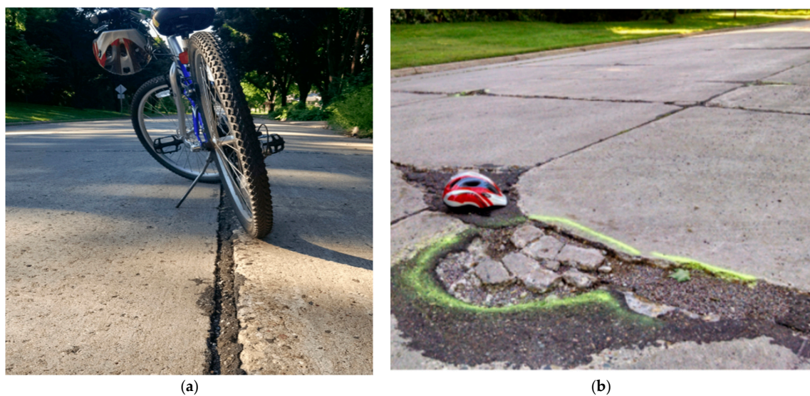
Figure 2. Examples of Rigid pavement distresses affecting bicyclists: (a) Faulting [4]; and (b) Spalling [4].
