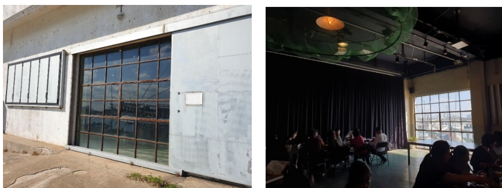
Figure 19. In order to save energy, insulation glass is placed, and natural light is employed for inside lighting (Source: Author's photo).
