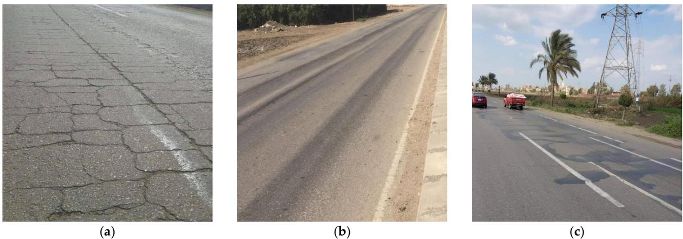
Figure 5. Block cracking on K-T highway (a), Rutting on K-B highway (b), and Bleeding in I-C highway (c).
