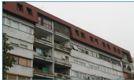
Figure 5. Appearance of the typical building in the settlement of ‘Konjarnik’ [87].
