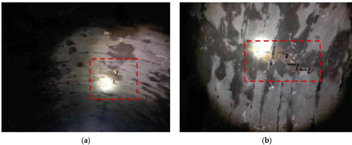
**Figure 8.** Cracking diagram of the lining of the right hole of the tunnel: (a) Peeling phenomenon of the primary support at the left vault of the right hole K142 + 115; (b) peeling of the initial branch at the left arch waist of the right hole K142 + 115.
