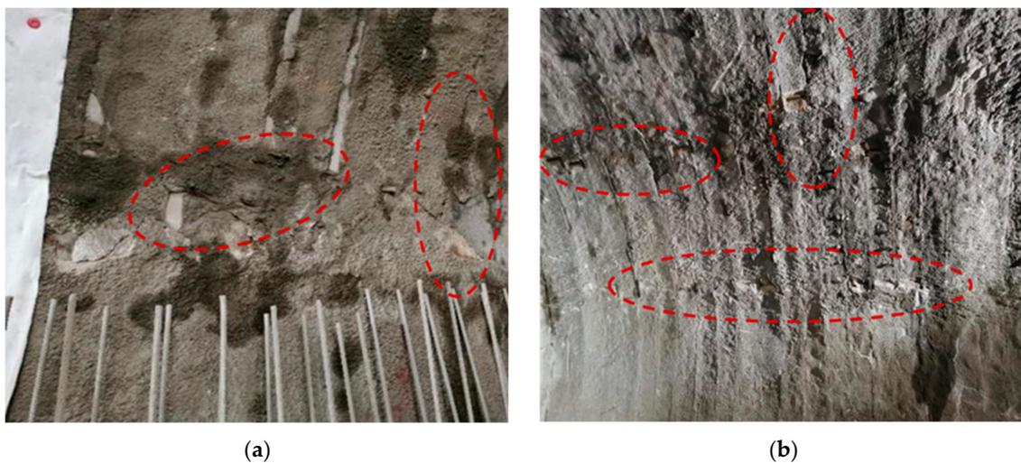
**Figure 9.** Cracking diagram of the lining of the left hole of the tunnel: (a) Cracks in the arch waist on the right side of the left hole ZK142 + 130–140; (b) cracks in the arch wall on the right side of the left hole ZK142 + 130–140.
