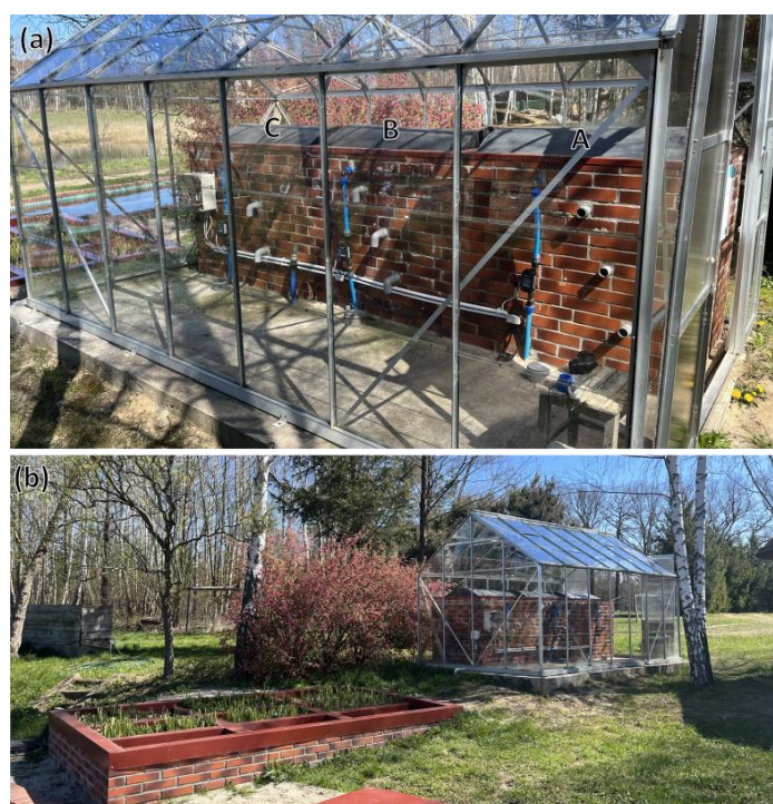
Figure 2. The NTSW pilot plant (adapted from Halicki and Halicki [13]). (a) Compost beds (A, B, C) in the greenhouse. (b) Installation of the whole NTSW pilot plant with part of the water renewal.
