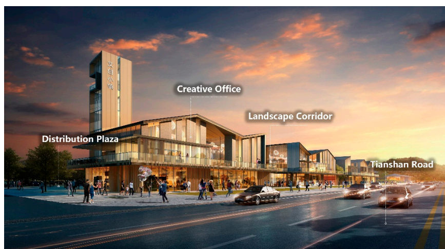
Figure 22. Jingmen Courtyard south district creative workshop.
