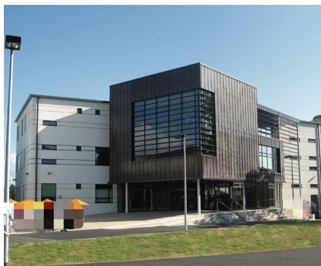
Figure 2. The building studied.
