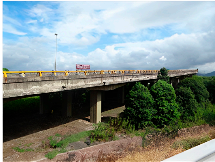
Figure 4. Image of bridge’s current state.
