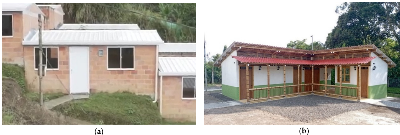
Figure 4. Photos of the houses under comparison: (a) CSB house (EDUR); (b) GaKB house at the UTP campus.
