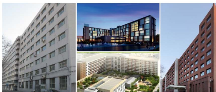
Figure 4. The picture on the left shows the original state of the building, the upper middle shows scheme F1, the lower middle shows scheme F2, and the right shows the final implementation, scheme F3.
