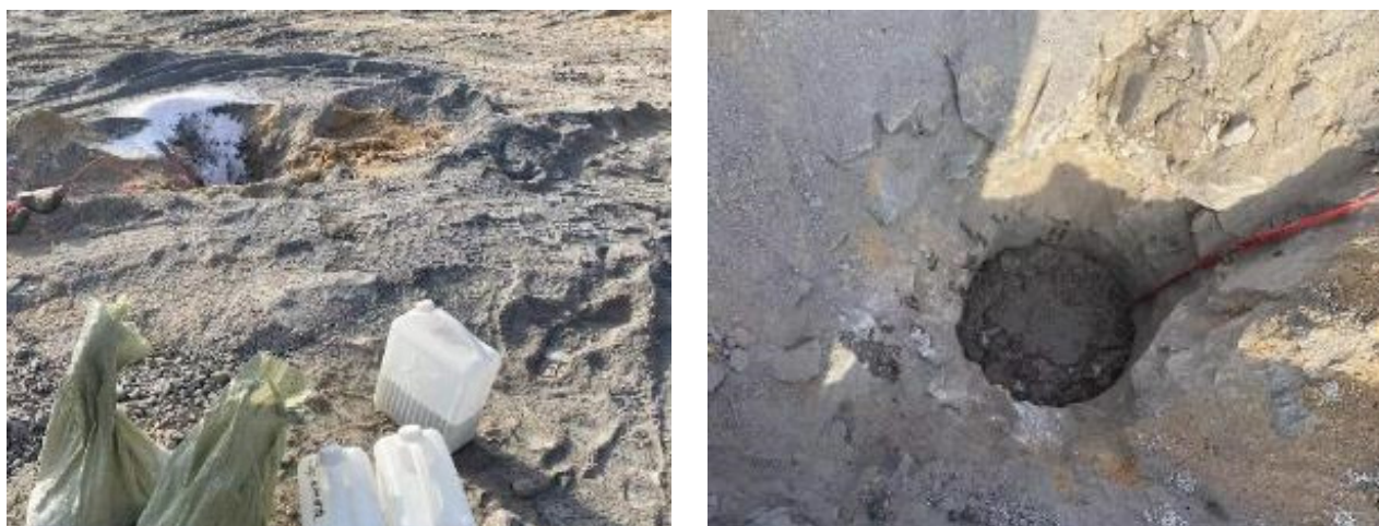
Figure 16. Blasting site operation construction.
