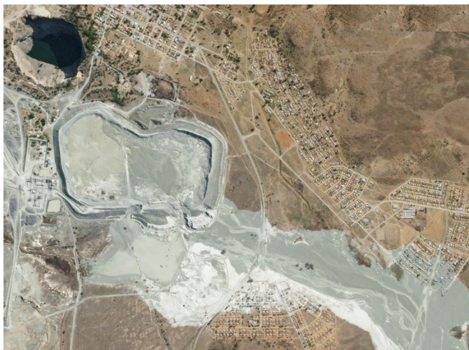
Figure 27. Jagersfontain tailings storage facility dam failure, 11 September 2022, South Africa.
