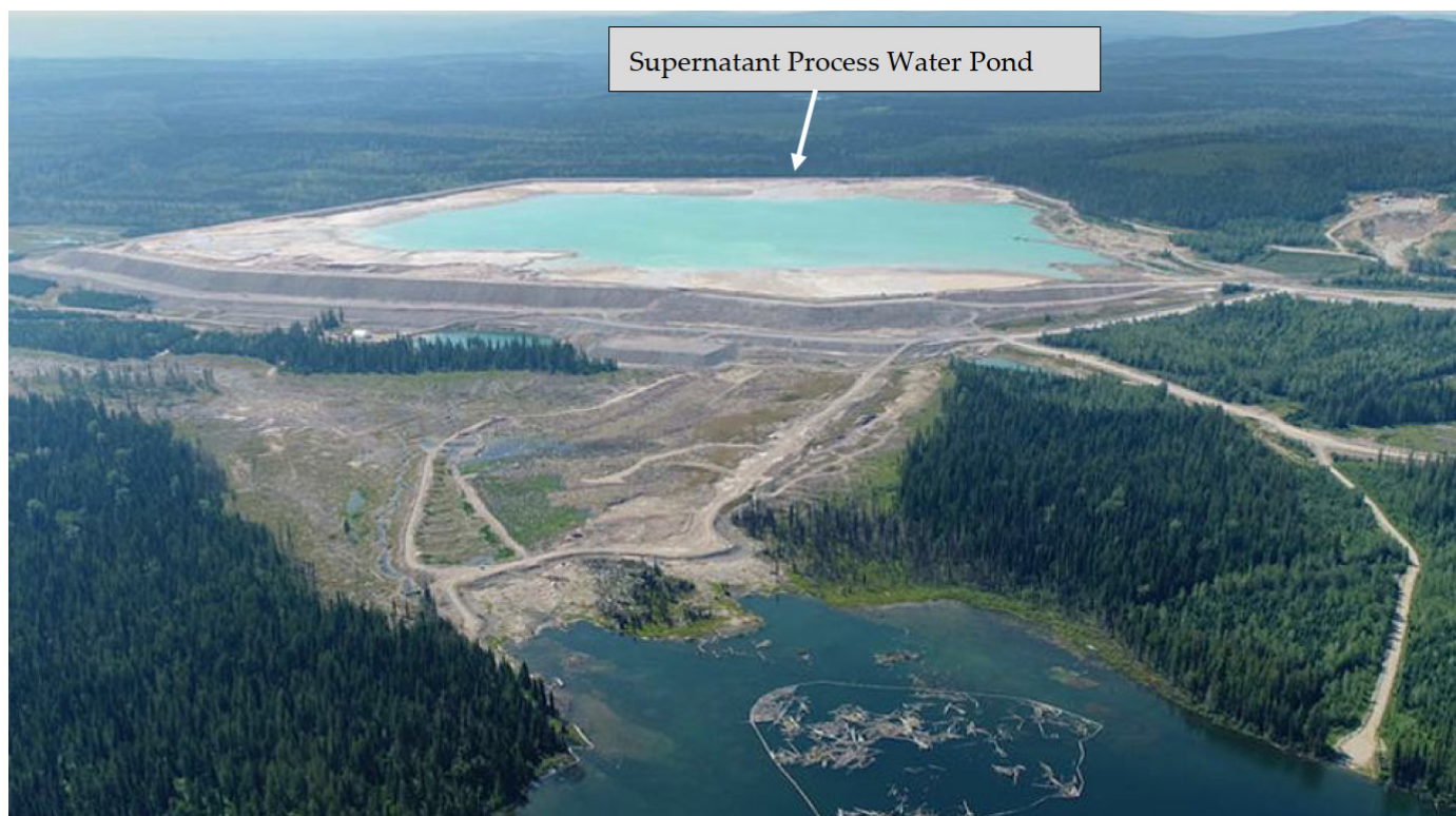
Figure 1. Mount Polley TSF—Canada, before the dam failure in 2014. The presence of a huge supernatant process water pond.
