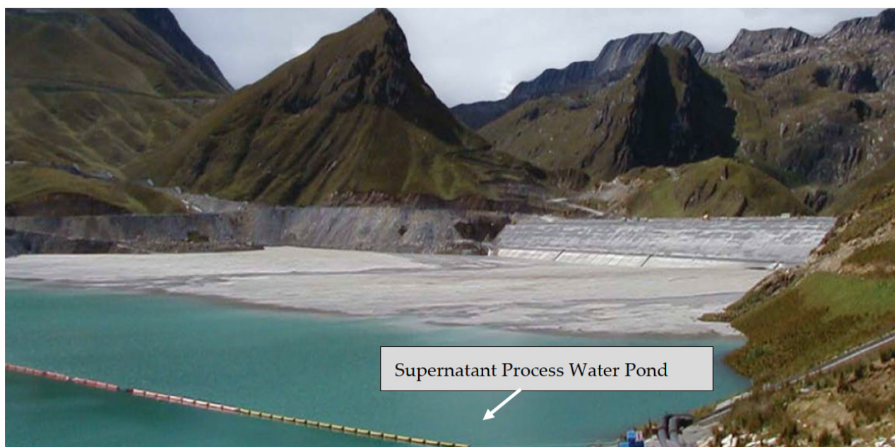
Figure 3. Example of panoramic view of tailings dam, tailings beach formation, and supernatant process water pond.
