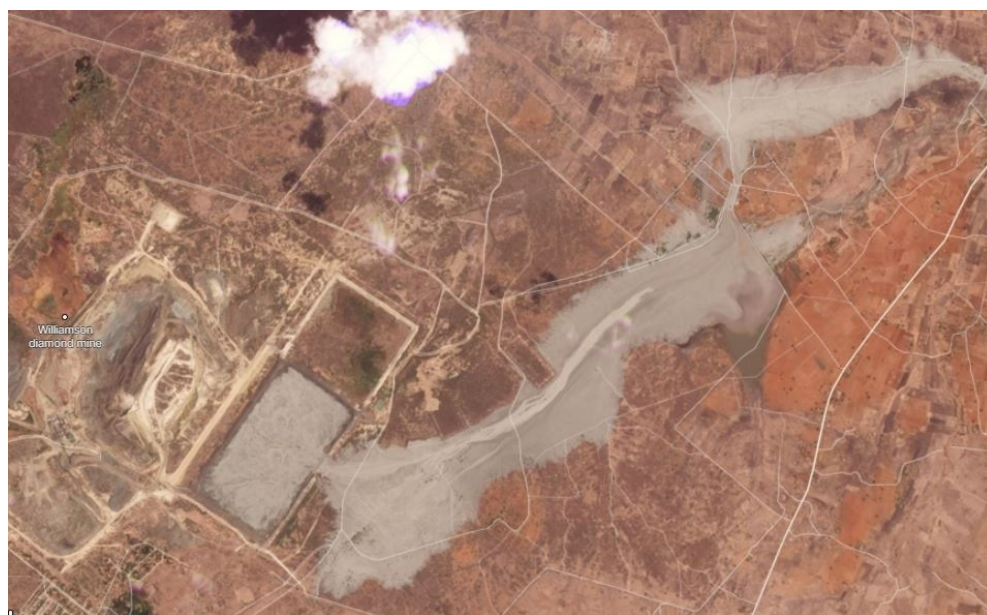
Figure 28. Williamson tailings storage facility dam failure, 7 November 2022, Tanzania.
