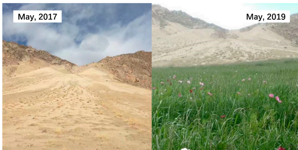
Figure 1. Comparison of restored and unrestored engineering slope at Gongga airport in Tibet.
