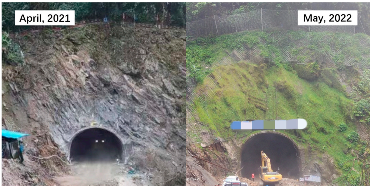
Figure 3. Comparison of restored and unrestored engineering slope at Laohuzui Tunnel entrance of Paimo Highway.
