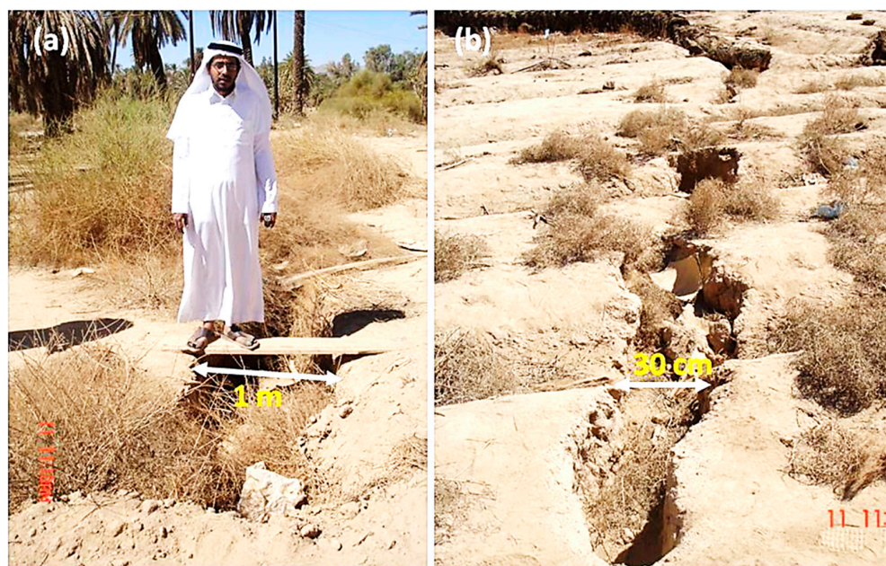
Figure 8. Fissures linked to subsidence because of groundwater over-withdrawal in Najran are shown in subfigures (a,b) in non-residence locations [2].
