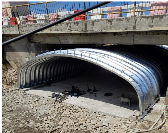
Figure 9. Steel structure connected with the foundation.
