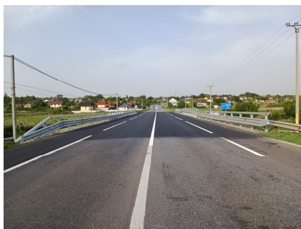
Figure 11. Global view of the bridge from the road surface.
