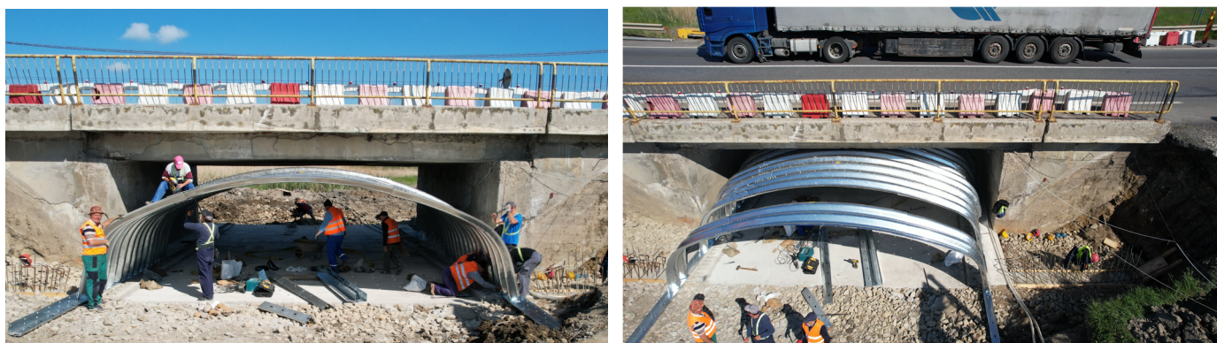
Figure 7. Photographs from the assembly process.
