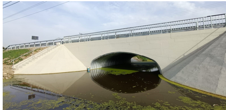
Figure 2. The finalized bridge.
