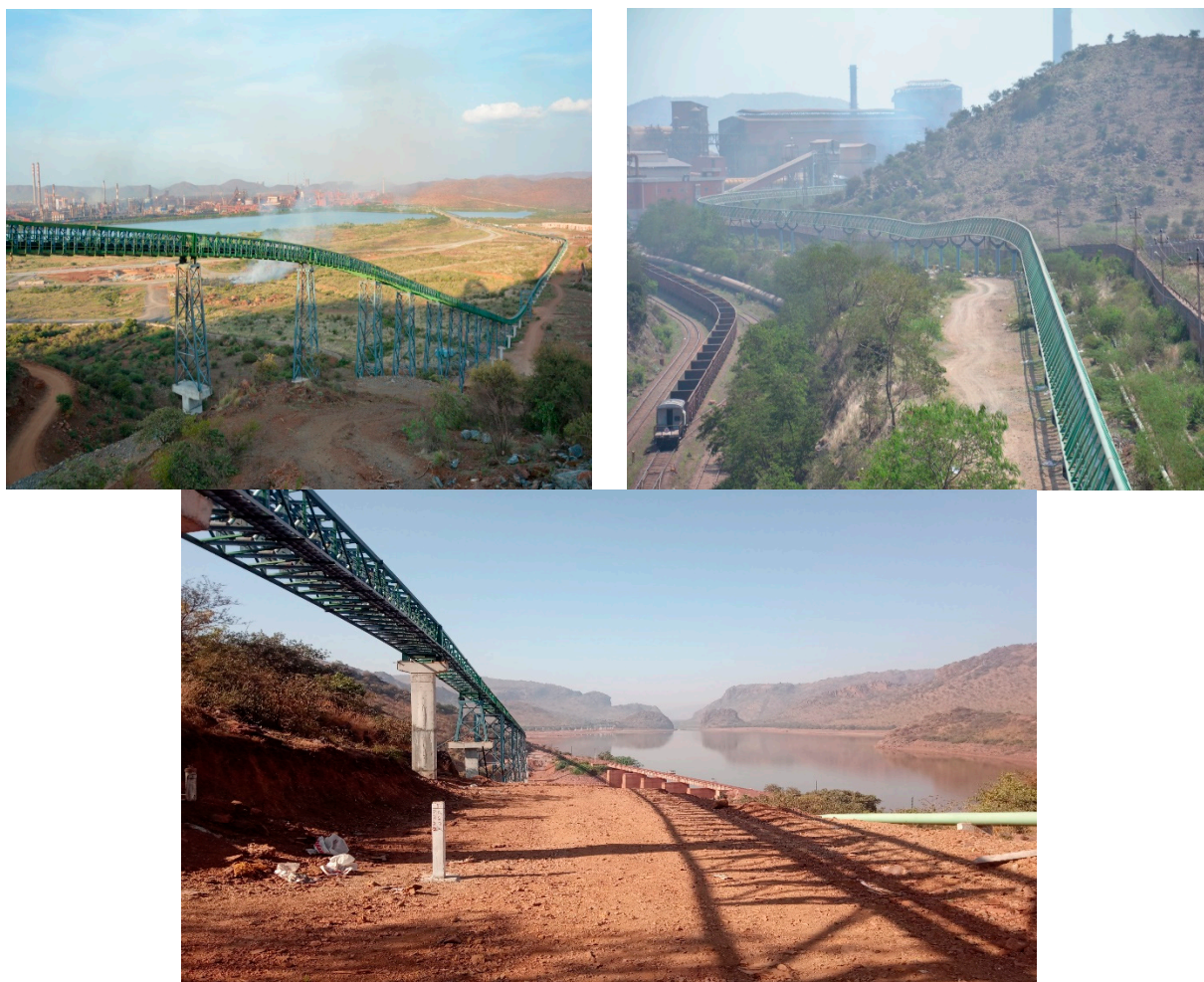
Figure 8. Closed pipe conveyor belt system used for transportation of iron ore.
