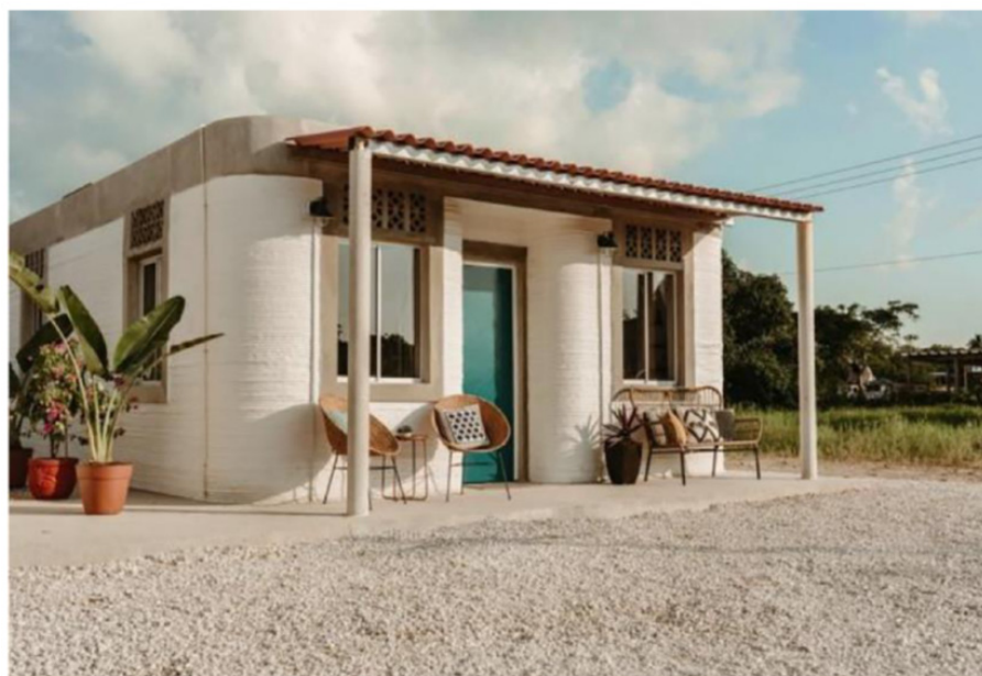
Figure 1. Example of one-story 3D printed construction (Source: [39]).
