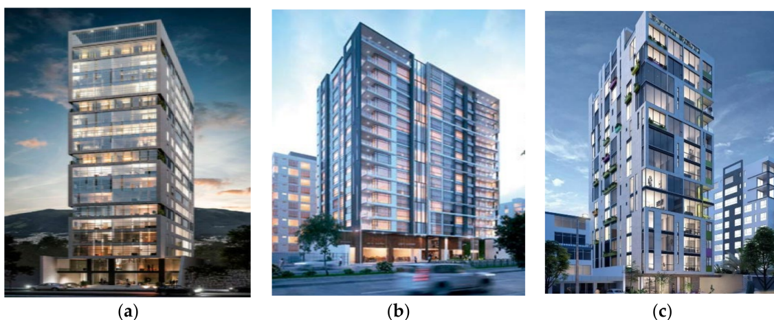
Figure 2. (a) Lafuente building; (b) Essence building; (c) Huma building.
