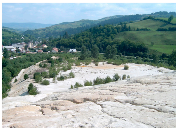
Figure 2. Gura Roşiei tailings dam, compartment no. 1.
