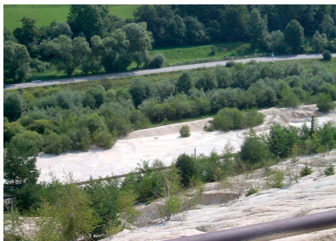
Figure 6. Gura Roșiei dam, waste retention compartments carried by rainwater.
