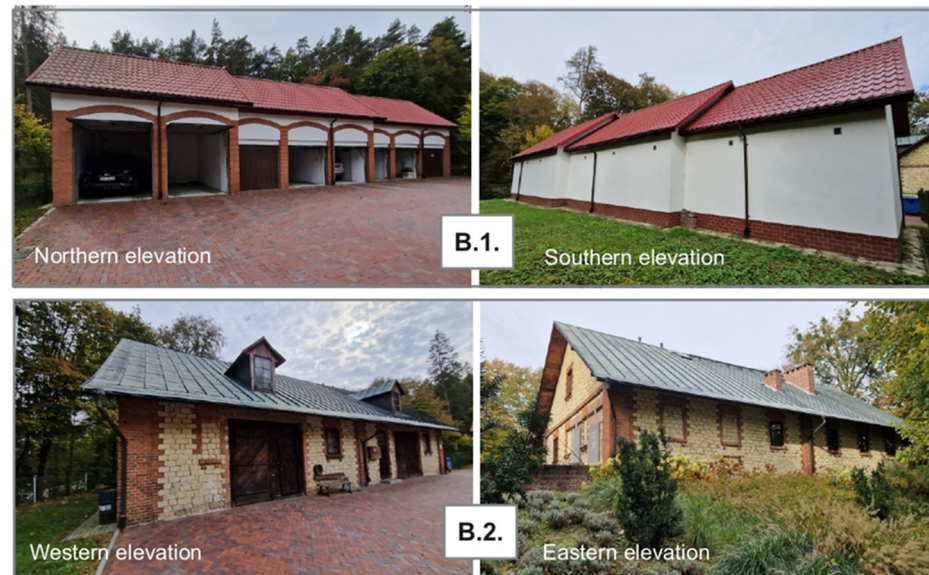
Figure 2. View of the garage (B1) and workshop (B2) in the Roztocze National Park Headquarters.
