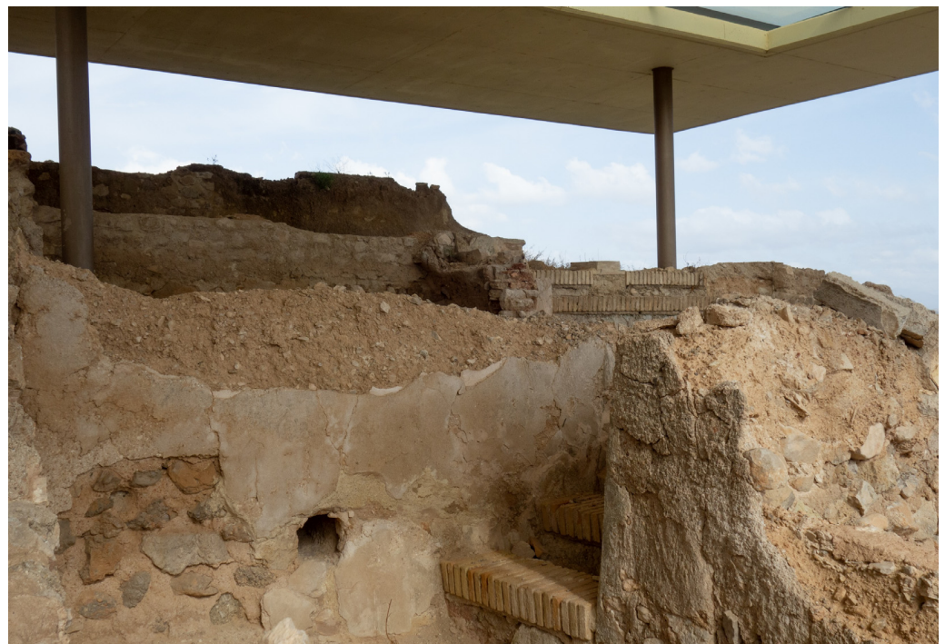
Figure 1. Partially collapsed rammed earth walls under contemporary protective cover at the archaeological site of Medina Siyasa (Cieza, Murcia).
