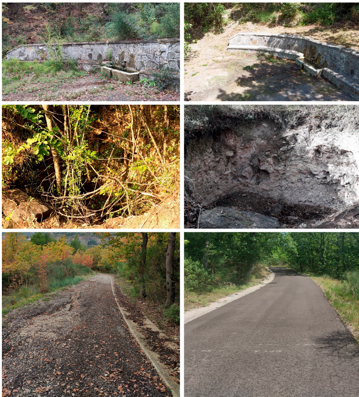
Figure 10. Pictures of the Kilns Trail taken during the survey campaign and the subsequent summer after maintenance work on the path and vegetation clearance. Top: maintenance work carried out at Fontana del Prato; center: vegetation clearing at one of the furnaces; bottom: restoration of damaged road surface (2023, © Authors).
