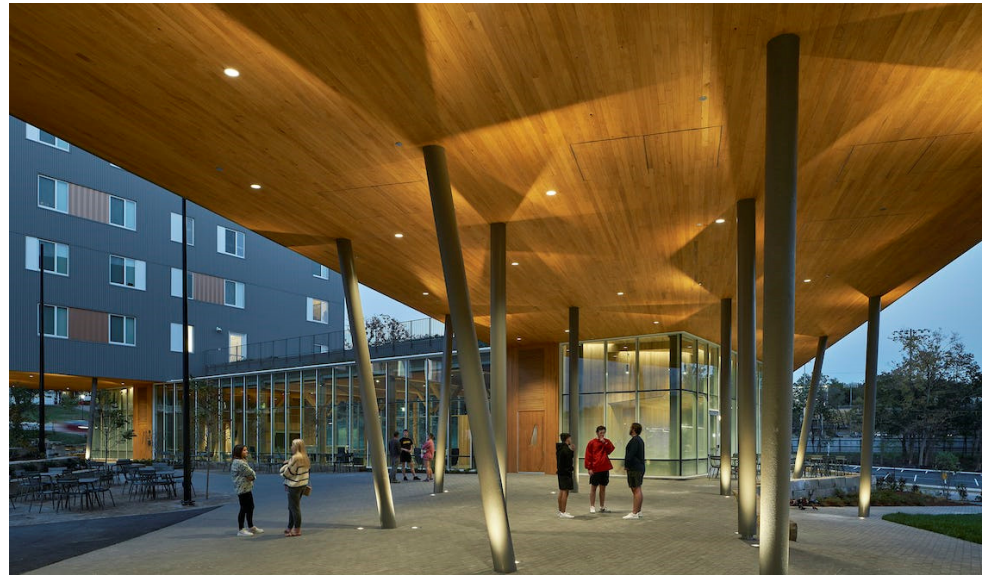
Figure 1. Adohi Hall, University of Arkansas campus, Fayetteville, AR (MODUS Studio).
