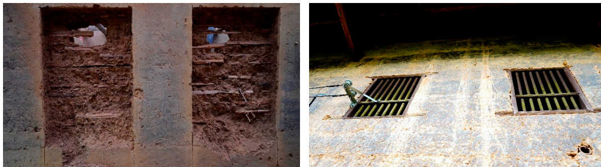
Figure 7. The internal structure of the earthen walls in the village's traditional rammed earth buildings shows remnants of the traditional formwork and scaffolding used in construction.
