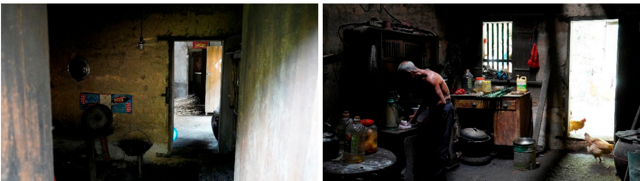
Figure 5. Interior condition of an existing rammed earth dwelling in the village.
