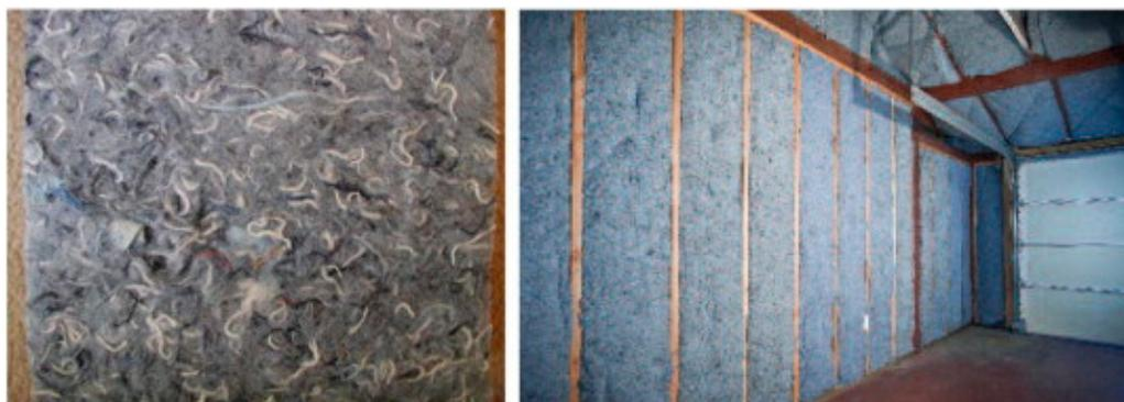
**Figure 15.** Recycled cotton for building panel insulation [20].
