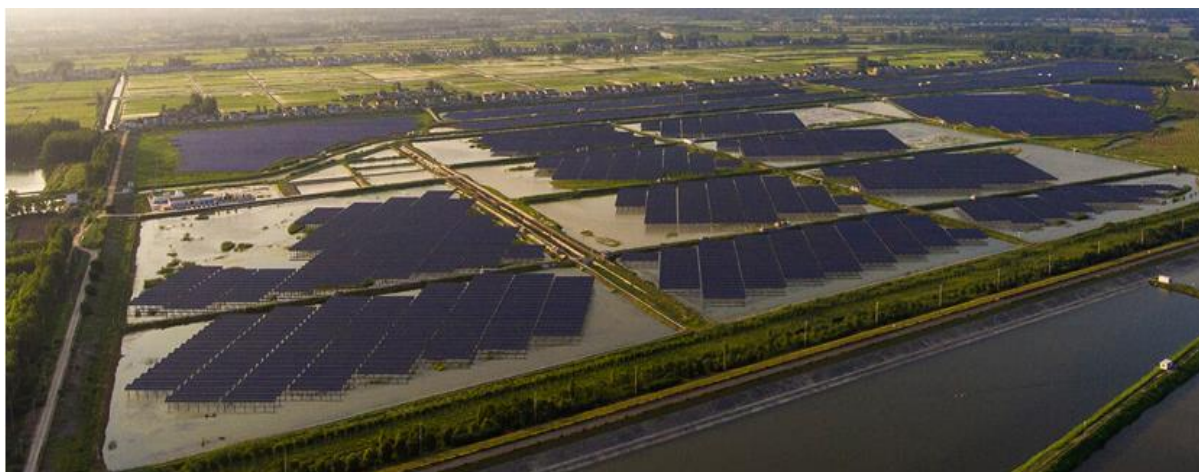
Figure 3. Overall layout of the TW “fishery–PV integration” base project.
