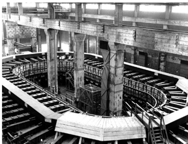
Figure 3. Picture of the Alpha Calutron track at the Y-12 Plant in Oak Ridge, TN, USA, that was used in part to perform U isotope separation for the Manhattan Project [35].
