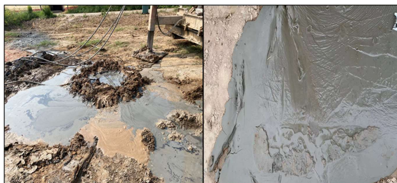
Figure 3. Slurry bubbling in conventional deep mixing techniques.
