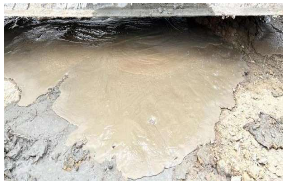
Figure 5. Slurry bubbling of DMJ pile techniques.
