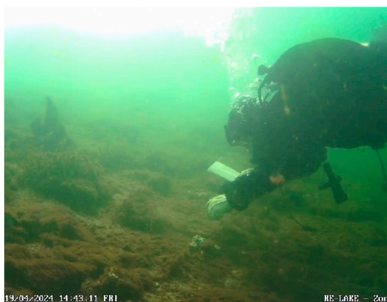
Figure 4. The underwater installation of different supports by a diver.
