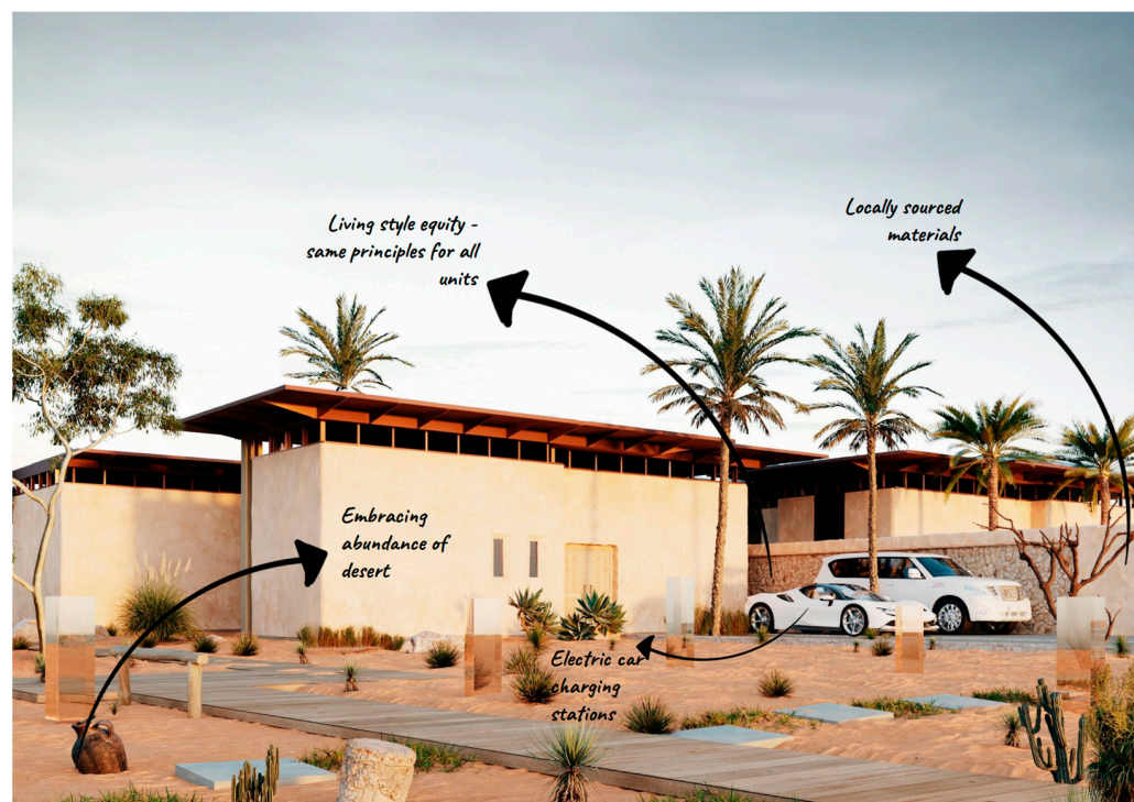
Figure 22. Unit SS—front view.
