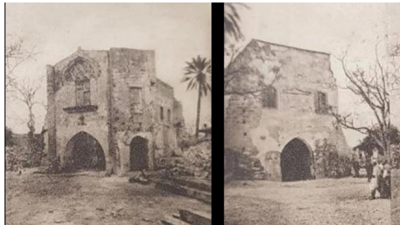
Figure 3. The front and back façades of the Lusignan Palace [6].
