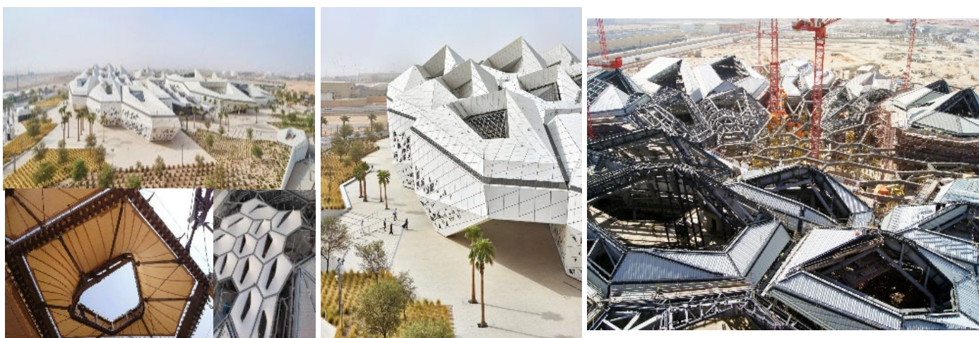
Figure 14. The KAPSARC's architectural design demonstrates a considered approach to environmental response, aligning with sun and wind patterns to optimize natural light, ventilation, and cooling. By adapting to the environmental conditions of the Riyadh Plateau, the KAPSARC reduces energy consumption and promotes a sustainable built environment. Source: KAPSARC—tensile fabric building skin.
