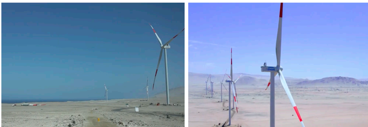
Figure 15. Panoramic view of wind turbines in the Punta Lomitas wind farm power plant.
