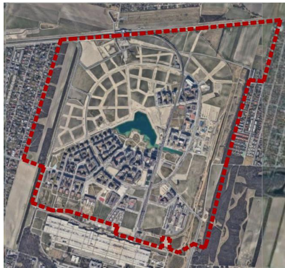
Figure 14. The borders of the Aspern Seestadt district. (marked red) The built and undeveloped areas of the SC project. Source: Original work based on a map from Google Maps.
