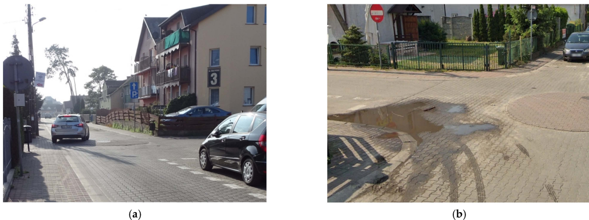
Figure 10. Traffic circle No. 2: (a) passages to the right of the central island, found to be the most frequent during the survey (source: own work); (b) image of the pavement after rainfall (source: Google Earth).
