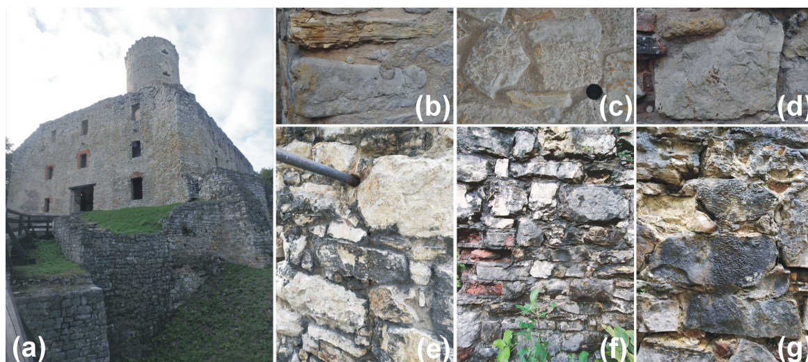
Figure 1. General view of the Lipowiec Castle after conservatory work in 2022–2023 (a). Examples of stones used for the construction of the castle, post-conservation: Triassic, wavy laminated limestone (b), Triassic organogenic dolomite (c), and ore-bearing dolomite (d). Signs of deterioration, black crust, and soiling on stone blocks and bricks before conservation (e–g).
